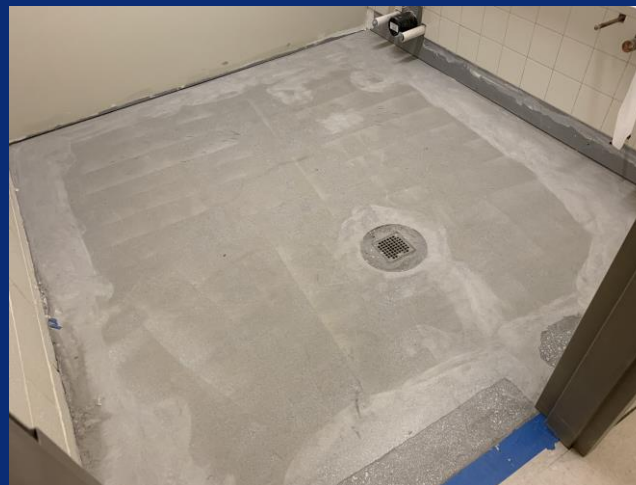
Floor Prep for Epoxy Flooring in Area C
